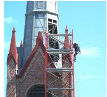
A steeple crew was brought in to re-skin the damaged area and to reinforce the framing to prevent future damage. The bulk of the cost of the repairs was covered by our insurance.
